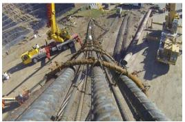
Figure 10: Two cranes lift over 100 feet of steel rebar pillars used in construction at the new Sanford Lab Homestake Visitor Center
